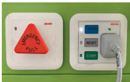
The workflow buttons can be assigned whatever workflow functions the hospital or other healthcare site wishes.
