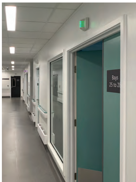
The system of overdoor lights at the new Chase Farm Hospital has proven especially beneficial, given that the 50-bedded inpatient ward is on a long corridor, with 42 individual en-suite rooms.
